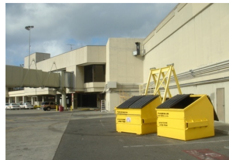
Figure 2. Typical trash bins located throughout ramp areas for use by State custodial staff, air carriers and ground handling companies.
