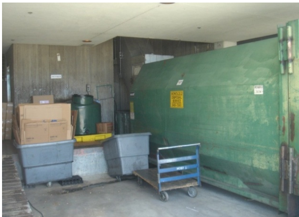
Figure 8. Example of a concession owned trash compactor on the ramp/apron level which helps manage waste capacity efficiently.
