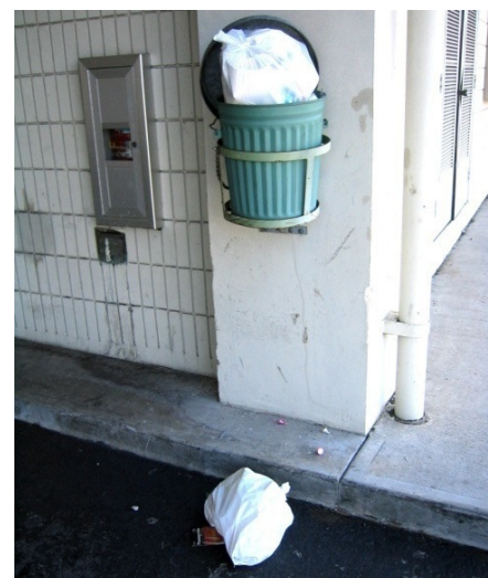
Figure 10. Protocol breached with trash bin lids ajar and trash not allowed to be left on the gate operations areas.
