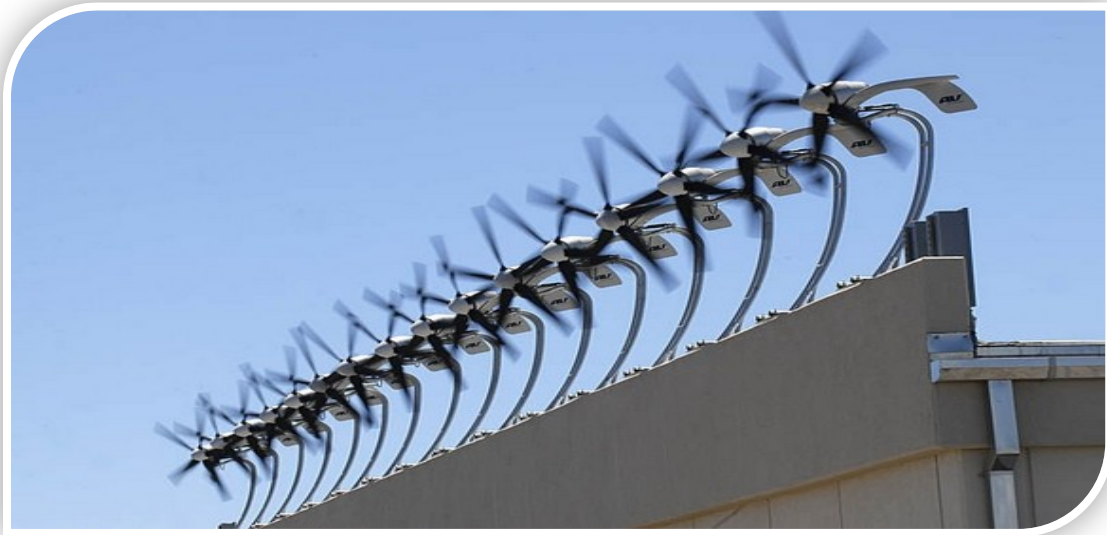
Above: A pilot wind energy project generates energy from the prevailing trade winds on an airport-owned building.
